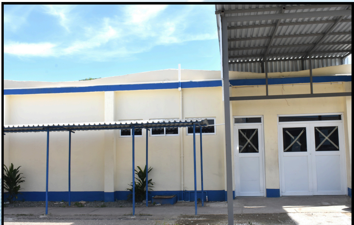
Image 2: Renovated Stores Building
