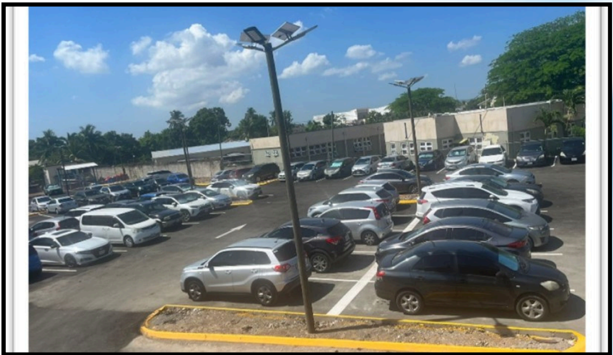
Image 1: Renovated Car Parking Lot
